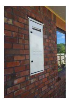
A recess box enables an external continuous flow water heater to be partially or fully recessed into an external wall, covered, and out of sight.
