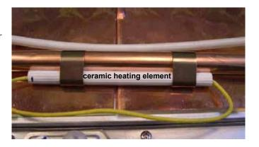
The heat, provided by strategically placed ceramic heating elements, stops the water from freezing within the pipework of the unit.
